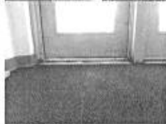
Typical Exterior Doors
